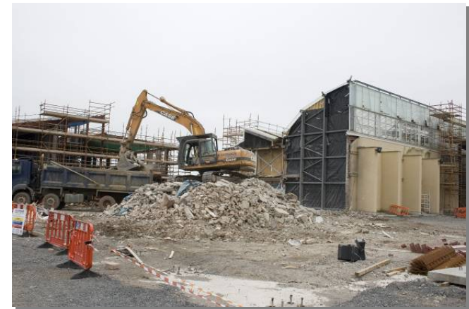
There has been good progress with the building over the summer.
